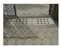
At the Rain Centre, the surface water flows to the gate. There is 3.5 feet long, 1 feet deep gutter with a reinforced concrete slab with holes. Inside the gutter there are pebbles. The cost of this gutter costs about Rs 600 per foot. A small bump on the roadside just next to the gutter can make sure that no water flows to the street.
