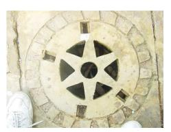
Percolation pit is used if enough space for a recharge well does not exist. The percolation pit is about 2' X 2' X 2'. There is a borewell with a PVC pipe of 6" diameter and 10 feet depth. In a large house, you can put a number of percolation pits all around house. The percolation pit at the centre cost Rs 1,500.
