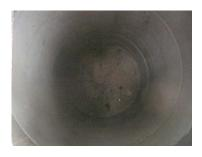
Water from the gate gutter is taken to the recharge well. The recharge well is 3 feet in diameter, 10 feet in depth. The purpose of the recharge well is to collect the vast amount of water collected quickly when it rains. The depth of the recharge well corresponds with the depth of the clay soil layer. There is no filter media inside the recharge well. If you already have a working well, try to direct the water from the gate to the well. The recharge well at the centre
