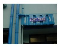
The loft tank is located at the first floor level. Water collected in this tank is used directly in the house using existing plumbing. The loft tank is made of PVC with a capacity of 200 litres. This particular loft tank costs about Rs 800. Water used for drinking and cooking must be boiled. Water supplied to the bathroom and toilets are used directly. A side benefit of rainwater is that it is soft water and hence will use less soap for cleaning purposes.
