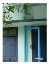
There are 3 drainpipes that bring the roof water down at the Rain Centre. These drainpipes are typically 3" diameter in size and capable of 6 Kg of water pressure. It costs about Rs 50 per feet installed (material + labour)
