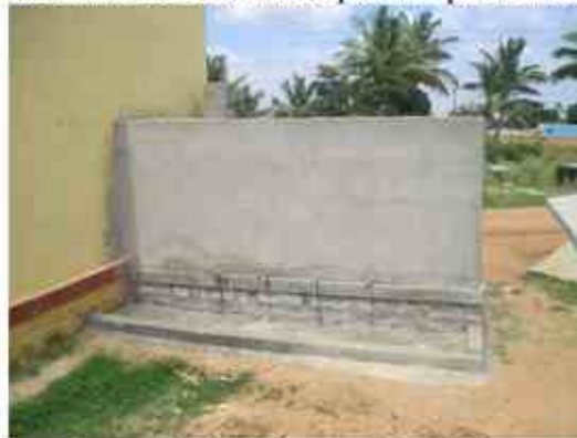
Fig 15: Cemented area below the tap for letting waste water out
