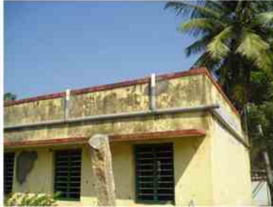
Fig 7: A well supported horizontal pipe for a flat roof
