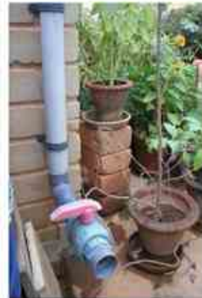
Fig 9 & 10: A good first rain separator with end cap on the wall Gate valve can also be used
