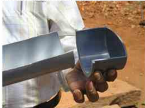
Fig 8: End cap for the gutter
