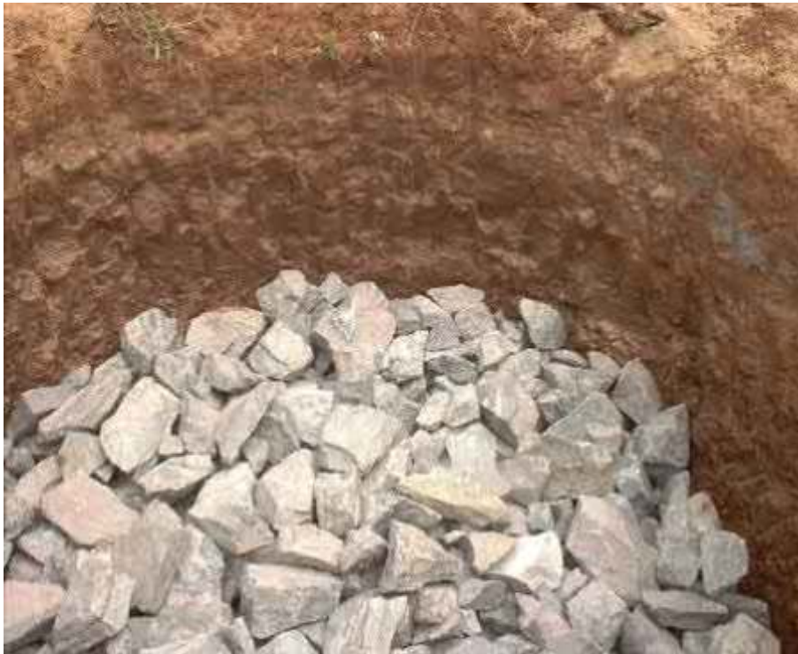
Backfilling. Round hard material.
