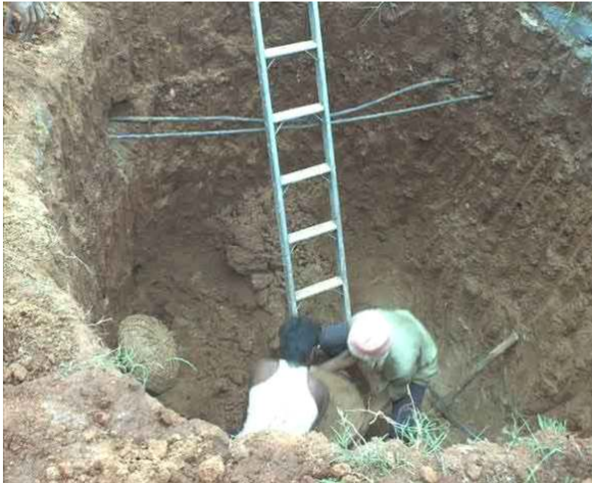
Digging the pit
