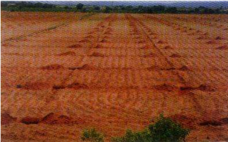
Lay out for pit digging
